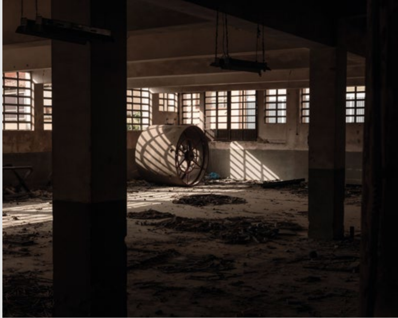
Inside the abandoned textile factory
